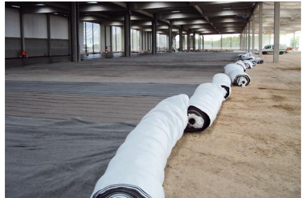
Figure 5. Installation of the geocomposite on the subgrade
