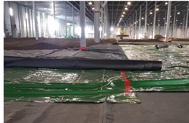
Figure 11. Vapor barrier and geotextile installation
