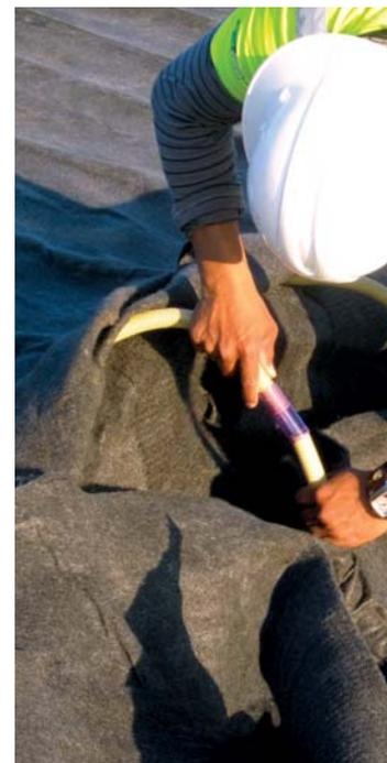
TOP PHOTO The tubular drainage geocomposite was deployed over the subgrade as a gas venting layer. BOTTOM LEFT Seaming of adjacent panels consisted of heat-bonding the geotextiles; no ties were needed. BOTTOM RIGHT At butt seams, the tubes were joined with mechanical couplers.
