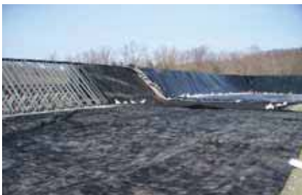
FIGURE 4 Above-ground impoundment for water storage.
