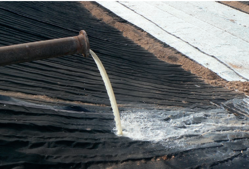
FIGURE 2 Multilinear drainage geocomposite used in a slurry dewatering facility. Photograph courtesy Afitex-Textel
