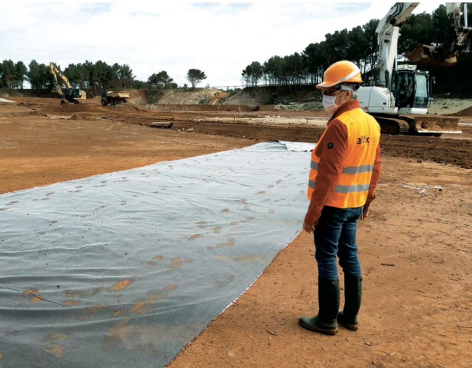
FIGURE 7 Installation of reinforcement geosynthetic
