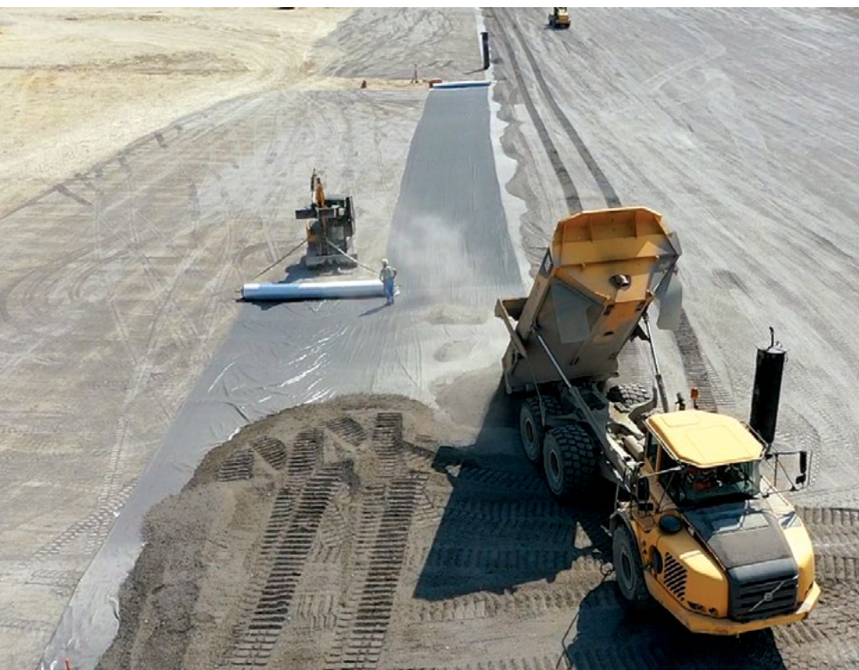
FIGURE 8 Placement of bottom ash soil over geosynthetic
