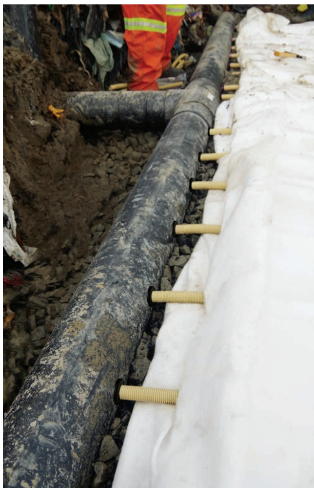
FIGURE 3 Connection of the minitube blanket to the collector pipe
