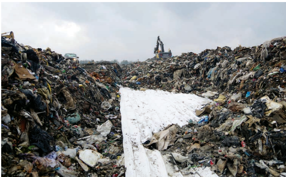
FIGURE 4 Backfilling with waste
