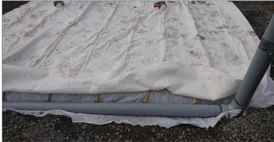
Figure 10: Connection to a collector pipe using Quick Connects
