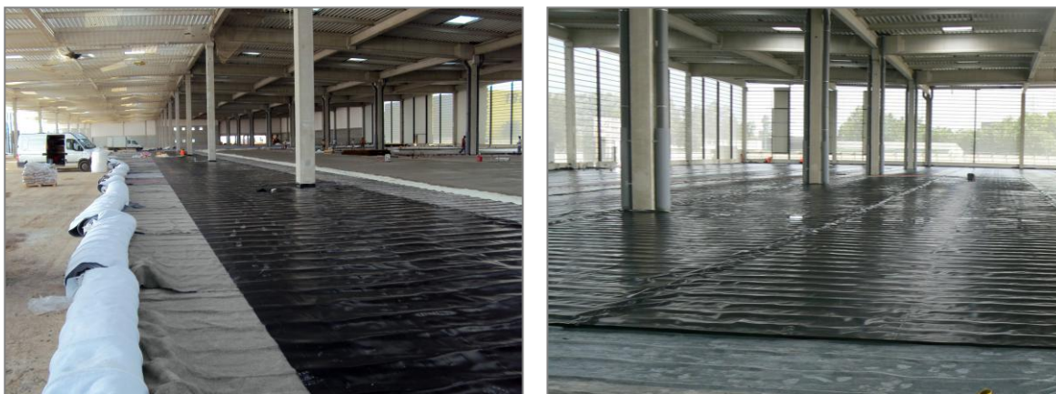
Figures 12: Upper geosynthetic layer placement
