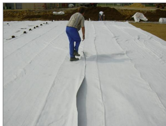
Figure 5: Side by side connections
