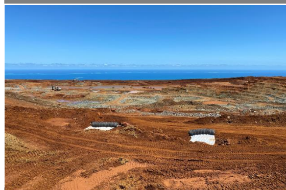
Backfill of DRAINTUBE 300P FT4 D25.
