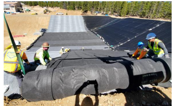
DRAINTUBE® installation on the slope. The product is light and flexible making it easy to install.
